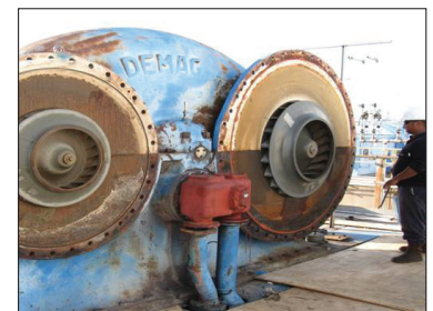
Maintenance of a Demag Integral Compressor
